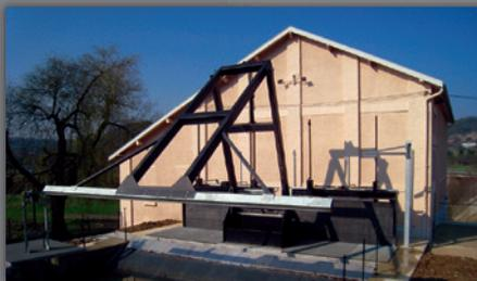
Fixed trash rack cleaner with channel discharge (fish friendly)
