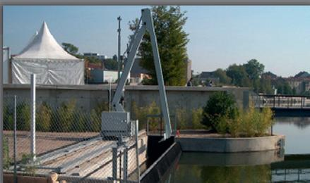
Travelling trash rack cleaner with channel discharge
